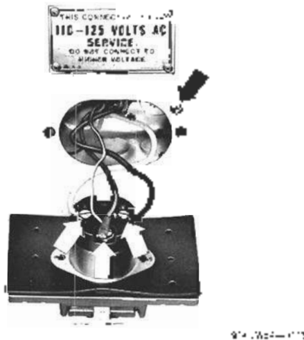
Fig. 7-6. Screw and wires that hold receptacle.
