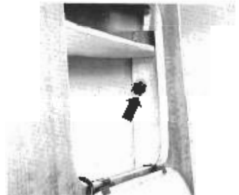
Fig. 7-12. Hand nut (arrow) at rear of closet.
