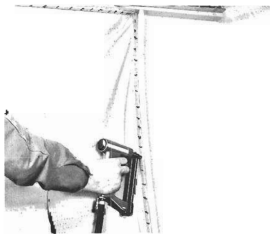
Fig. 7-38. Staple gun being used to attach the bellows and plastic strips to the wooden frame.
