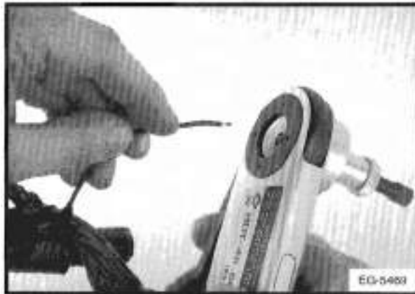
Figure 6-7. - Insert Wire Into Contact
