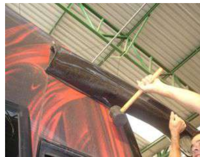
Use a rubber hammer to start the sliding movement
